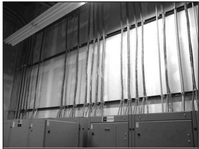
Figure 6.1—Installation of Type MC Cable (courtesy Braggs Electric Construction)
